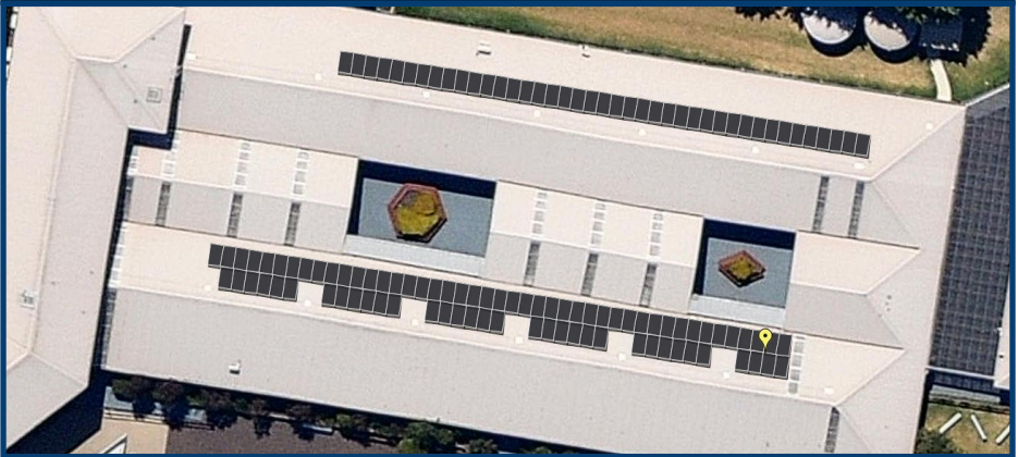
Solar Panels on BEAM Sub School Building
